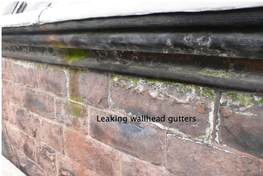
New cast iron rainwater goods to be provided
