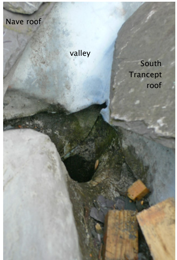
Rainwater outlet—to be increased in size
