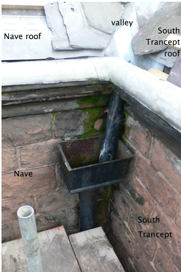
New cast iron rainwater goods to be provided
