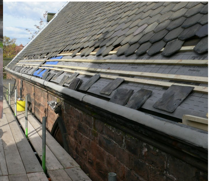
3 courses of slates stripped from South side of Nave roof and West side of South Trancept roof prior to gutter repairs
